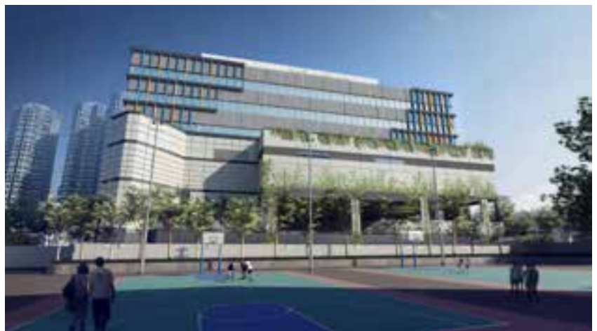
New Territories West Regional Officer and Water Resources Education Centre of Water Supplies Department, Tin Shui Wai Client : Architectural Services Department Project Period : Aug 2015 to Feb 2018
