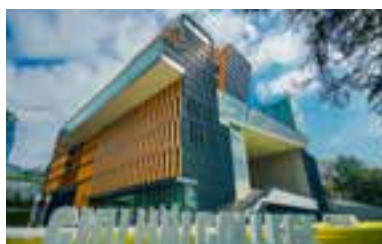
▲ Main Contract for Campus Development of Chu Hai College of Higher Education
