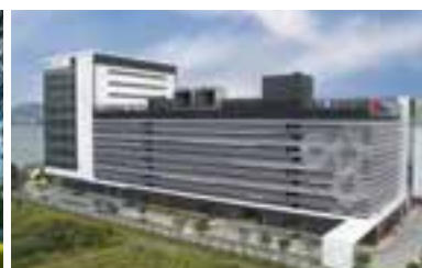
▲ Main Contract for Sub-Structure and Superstructure for the Proposed China Unicom (Hong Kong) Global Center
