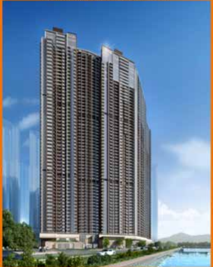
Residential Development at Lohas Park Package 6
