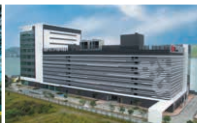
▲ Main Contract for Sub-Structure and Superstructure for the Proposed China Unicom (Hong Kong) Global Center
